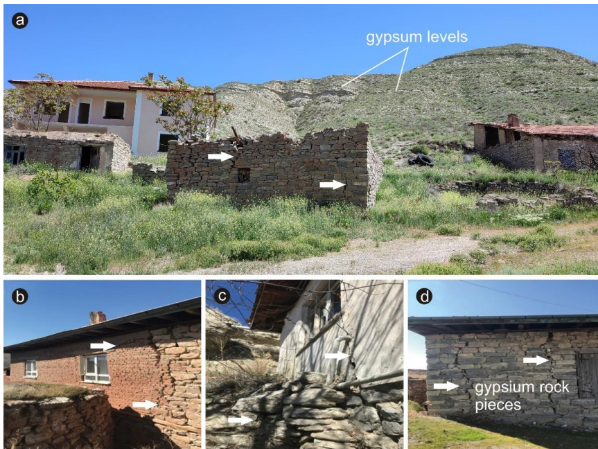
Figure 4. (a) Gypsum levels and buildings from study area; (b,c,d) Images of damaged buildings from the study area [11].
