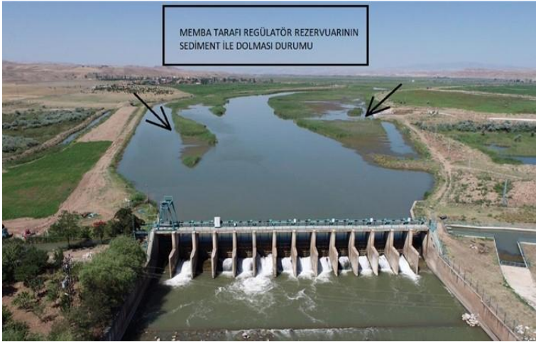
Figure 2. Surface view of sediment accumulation of the reservoir in front of the regulator in the study area [5].
