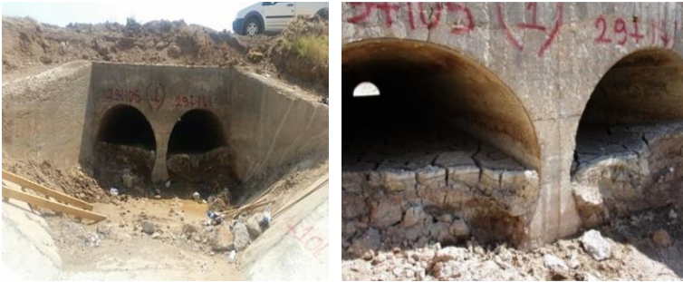
Figure 3. The situation of the area where the water passage should be made in the study area as a result of sediment accumulation [5].
